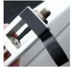
After installing any necessary linoleum shims, wrap electrical tape around the mount carefully. If you have a lot of snow and highly corrosive con-ditions, wrap all open spaces with tape also.
